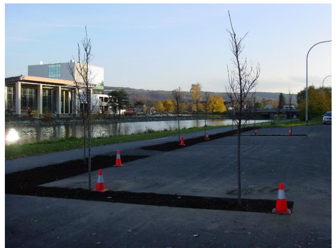
The finished parking lot
