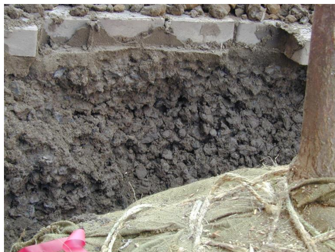
Closeup of CU-Structural Soil® after installation
