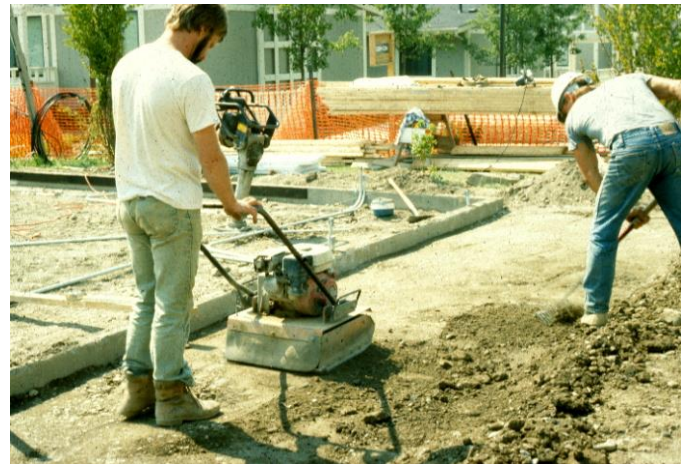
Compaction of soil in preparation for pavement
