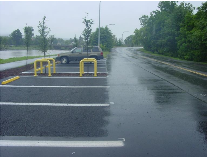
A porous asphalt and CU-Soil® installation in Ithaca, NY just after construction
