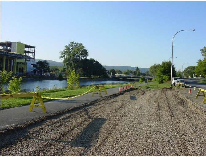
CU Structural Soil® was used as a 2' deep base course for the entire parking lot
