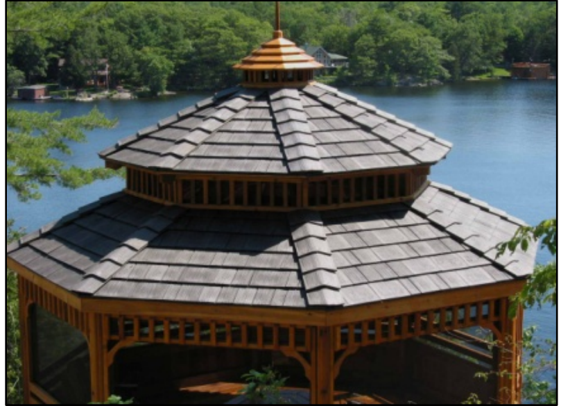
Enviroshake gazebo roof
