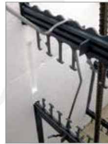
Vertical Clips in Place
