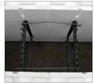
Horizontal Clips in Place
