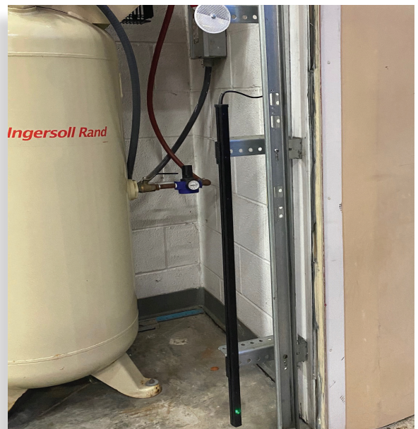
Miller Edge Monitored Light Curtain (MLC-K36) installed in multiple apparatus bays at the Winchester Kentucky Fire Department
