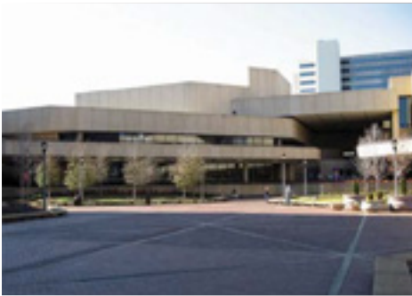
Birmingham Jefferson Civic Center Birmingham, Alabama
