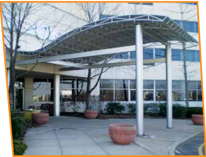
Completed back entrance
