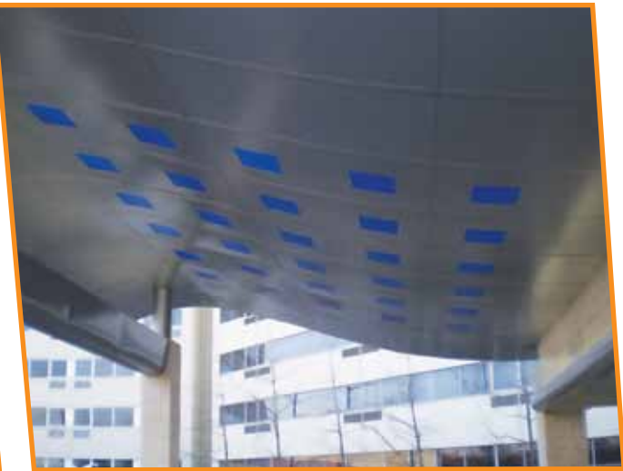
Front entrance – canopy interior close up
