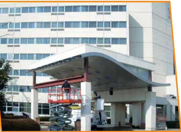
Installation of Front Entrance
