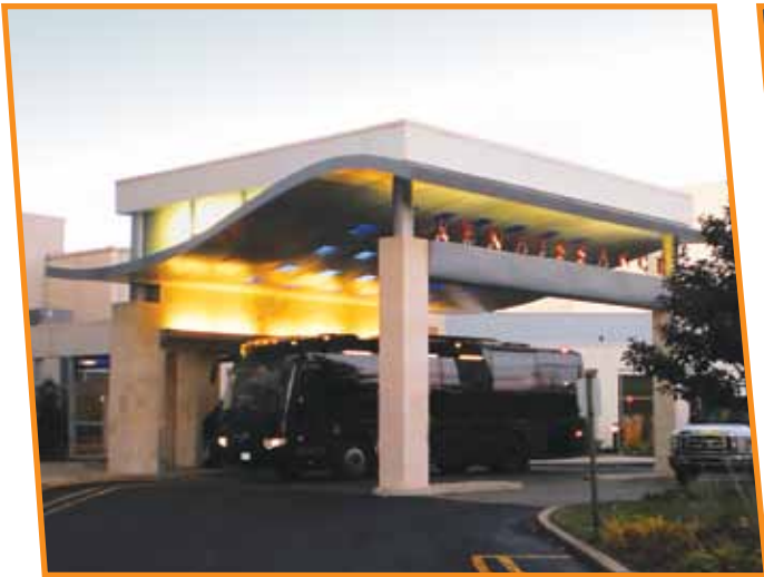
Completed front entrance
