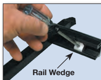
Tightening rail wedge on shortened section.
