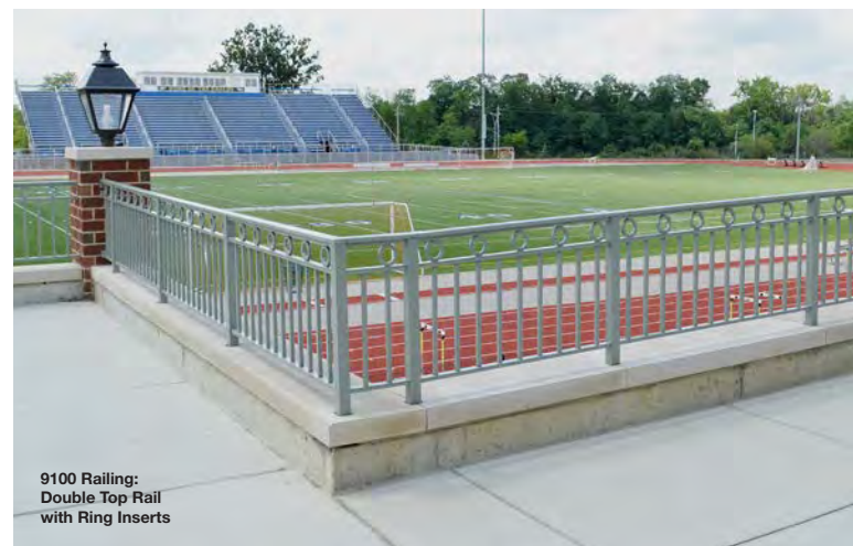
9100 Railing: Double Top Rail with Ring Inserts Side Mounted on a Rooftop
