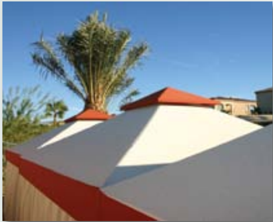
Roof Top Air Vent
