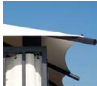
Rafter and roof-line of the Polynesian Cabana, painted steel frame and fabric roof membrane.
