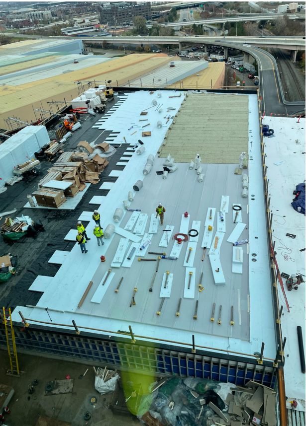
Needed mineral wool being installed
