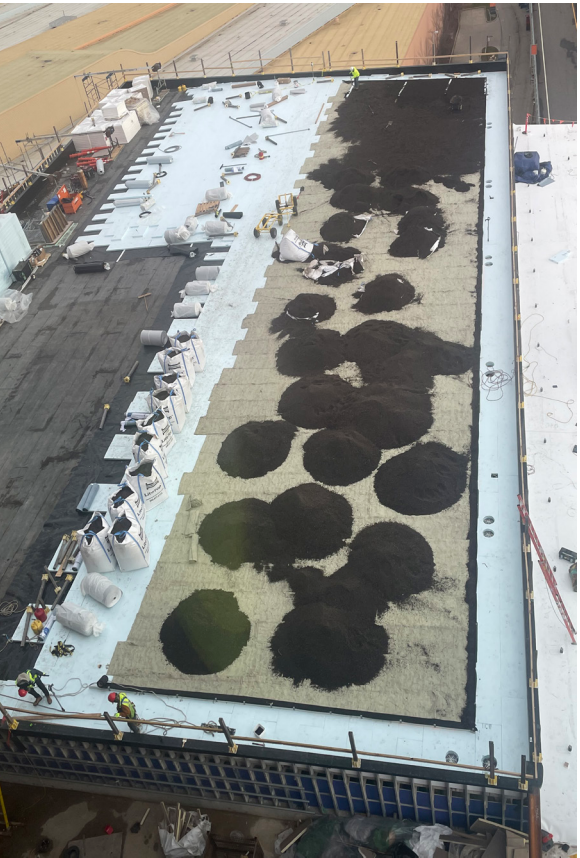
Growing media being installed
