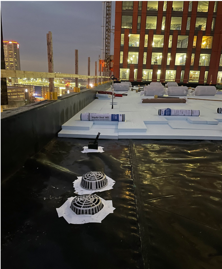
Root barrier and insulation layers being installed
