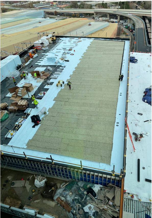
Needed mineral wool installed
