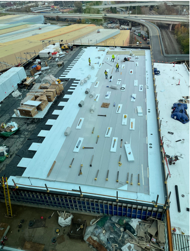
Detention layer being installed
