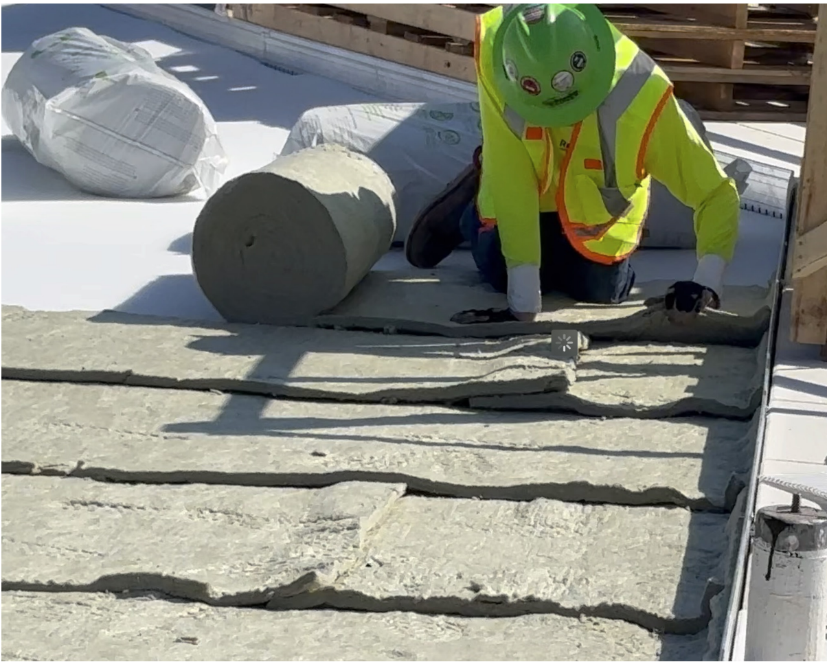
Needed mineral wool being installed
