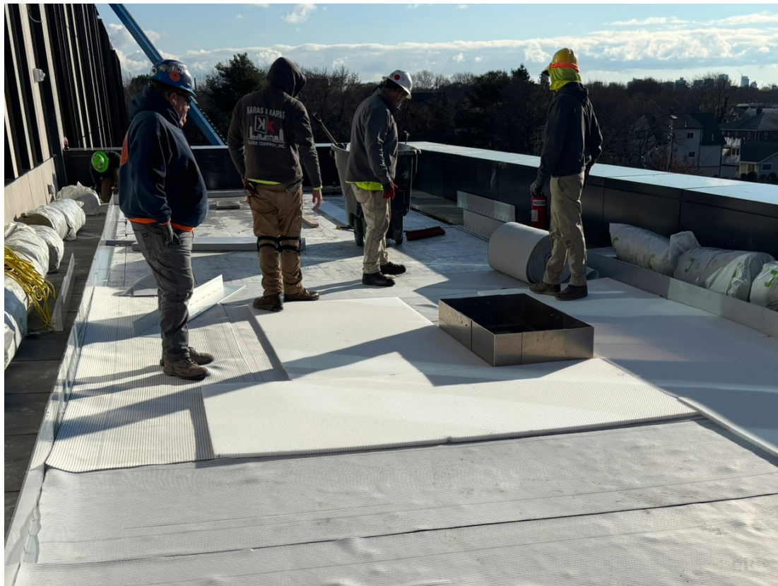
Drain Enclosure installad at roof drain
