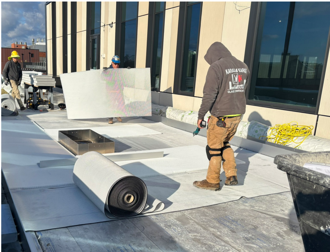
Detention Layer installation
