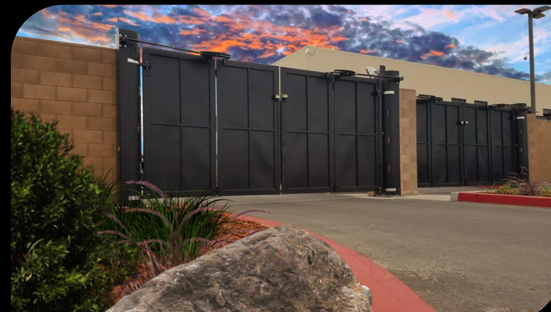
High Speed, Solid Panel Police Headquarters Installation
