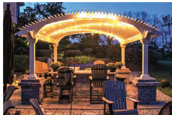
14'X18' ARCADIAN Standard Unit installed on Footers
