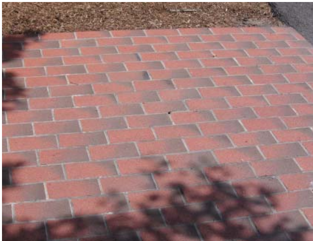
Photo 1 Clay Pavers in a Mortar Setting Bed
