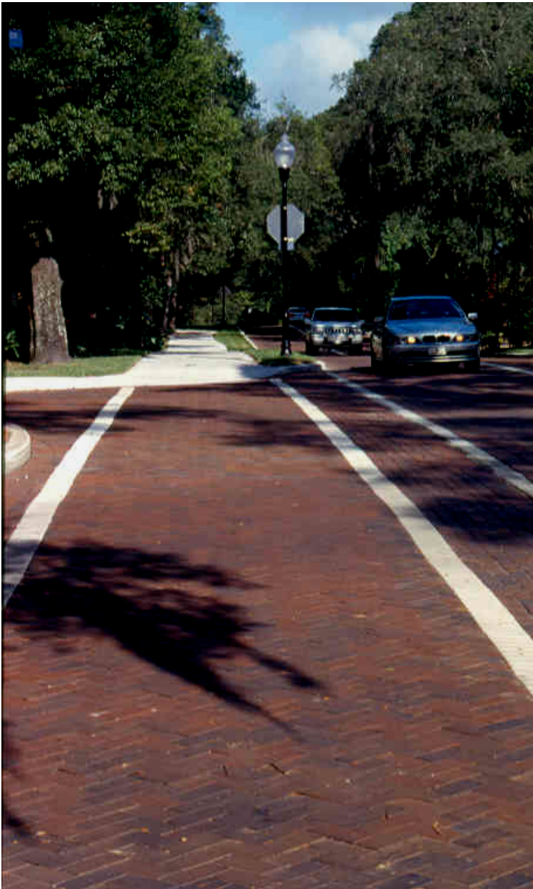
New Traffic Calming Clay Pavers
