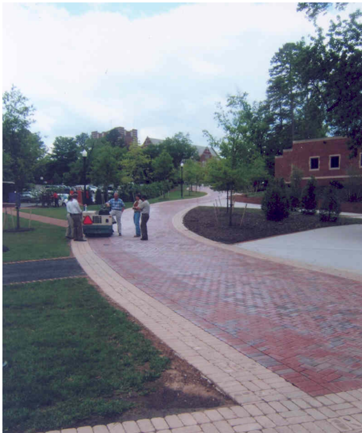
Picture: Efflorescence Vacuum
