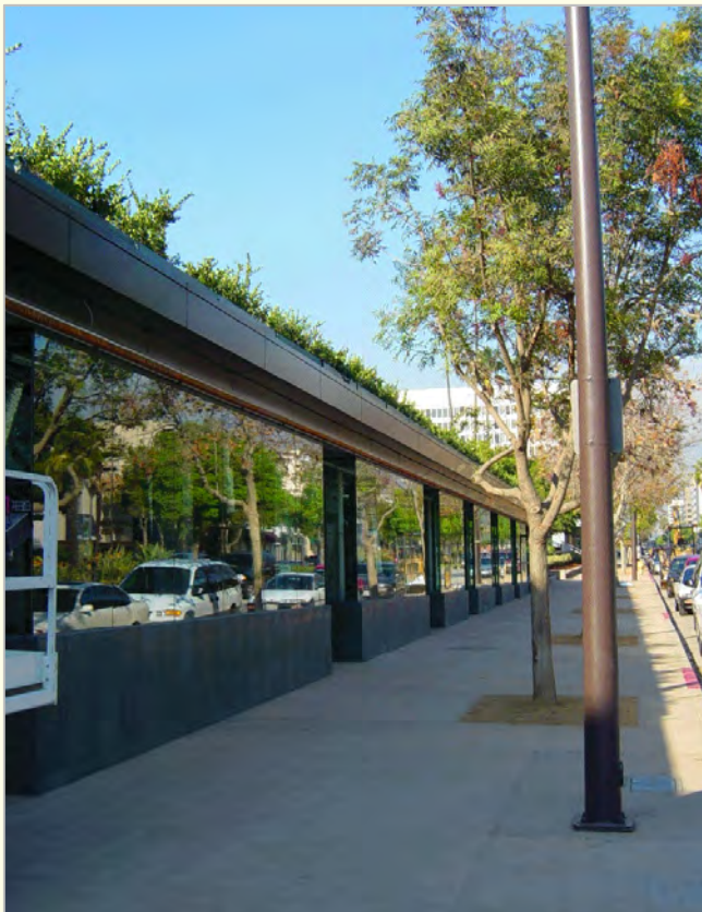
Roof Top Planters in Pasadena, California
