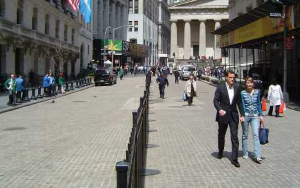
▲ New York Stock Exchange Streetscape+Security Project, New York, NY: MILANO GRANDE grey mix porphyry Quennell Rothschild & Partners LLP / Rogers Marvel Architects, LLP
