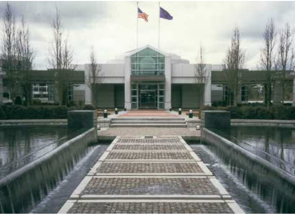
▲ Nike World Campus, Beaverton, OR: MILANO grey mix porphyry OTAK, Landscape Architects
