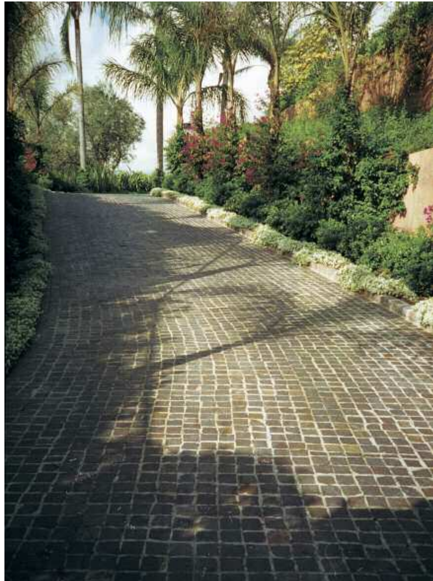
▲ Residence, Beverly Hills, CA: Serpentine Drive FIRENZE + MILANO GRANDE red mix porphyry
