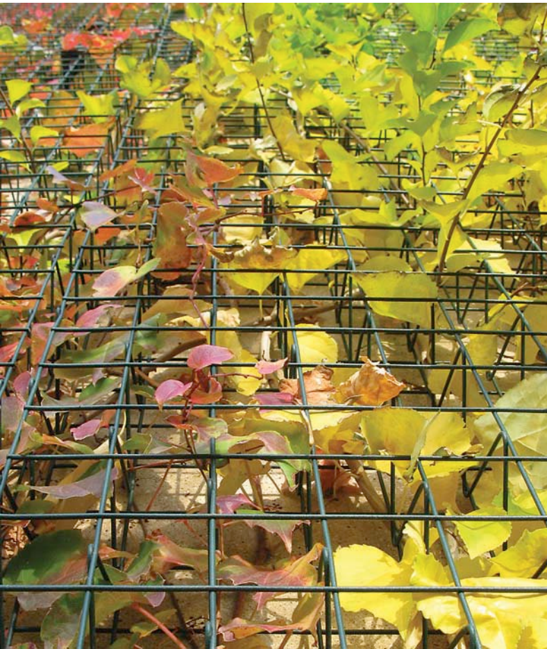
A wall mounted, modular, three-dimensional, green facade system with plants showing seasonal interest, Chicago, IL
