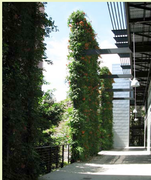
Green facade technology can create shade that cools building surfaces, and also provides privacy screening
