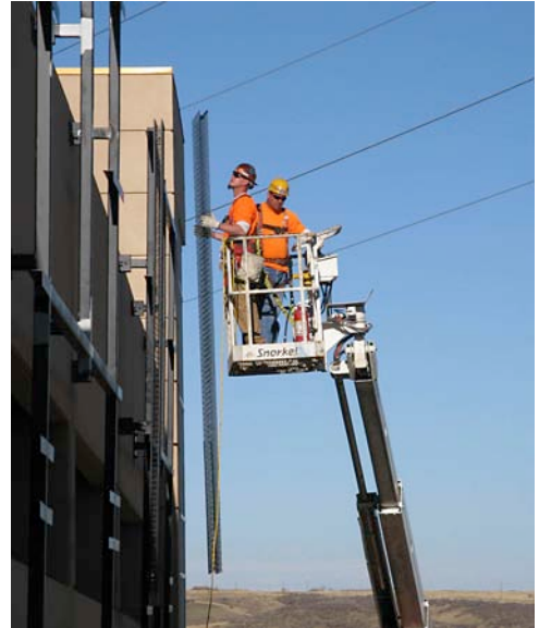
Rigid, lightweight, three-dimensional panels being installed on a multilevel building, Golden, CO
