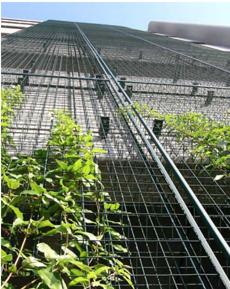
Six story green facade with three-dimensional panels engineered for wind and snow loads, Rockville, MD
