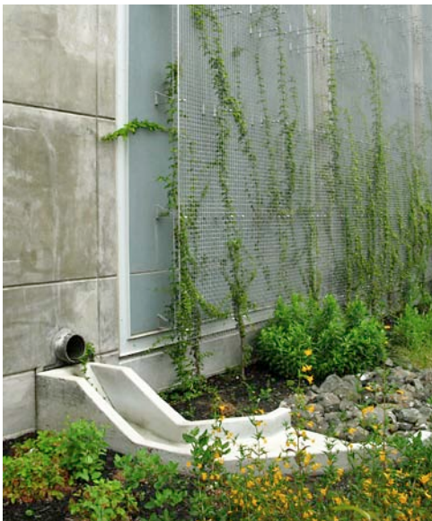
This rain garden with integrated green facade is a key component to the stormwater management strategy, Oakland, CA
