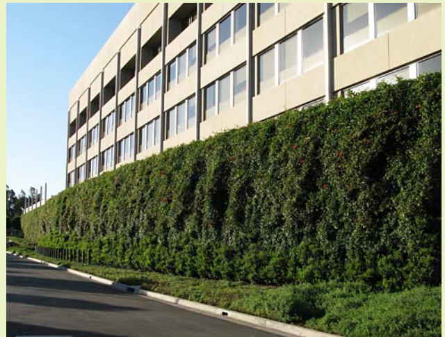
300 feet of freestanding green facade provides security, shade and privacy screening, Irvine, CA
