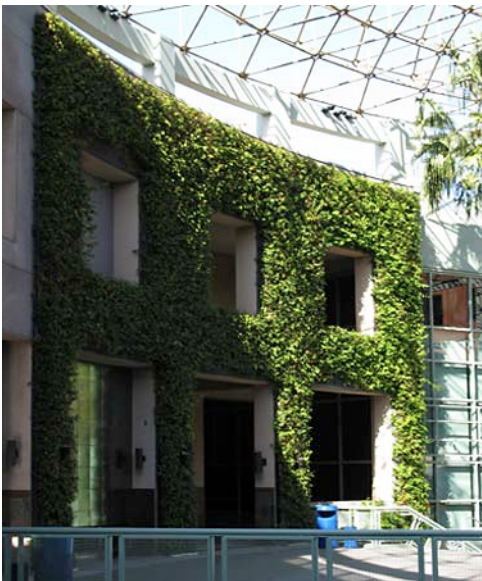
Proper soil volume, irrigation delivery and maintenance are successfully demonstrated in this 18 year old green facade installation, Universal City, CA
